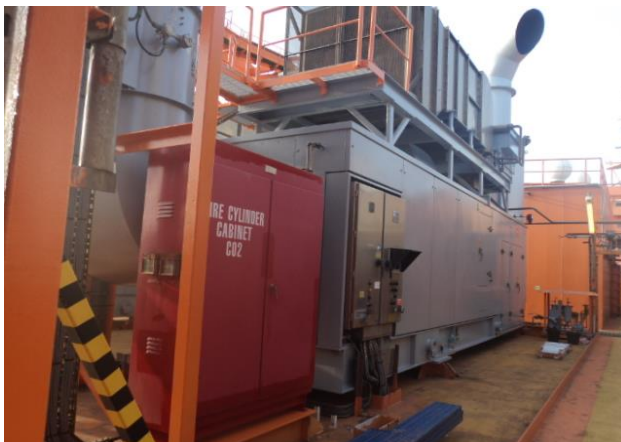
After final coat on solar in U-70
