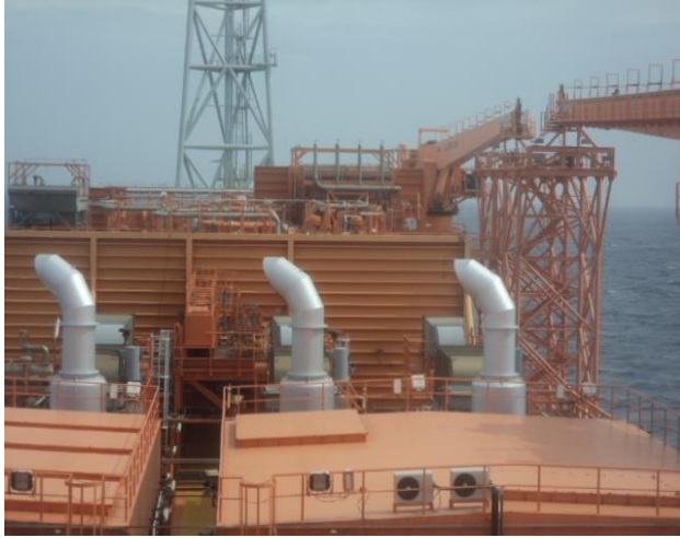
After final coat in U-20 & solar area
