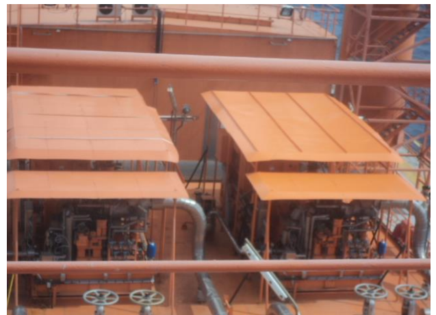
After final coat in U-10
