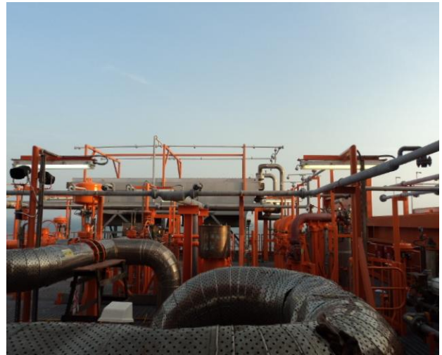
After final coat in P-10 top side
