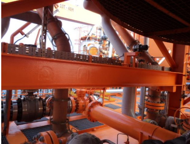
After final coat on top side of gas compressor area
