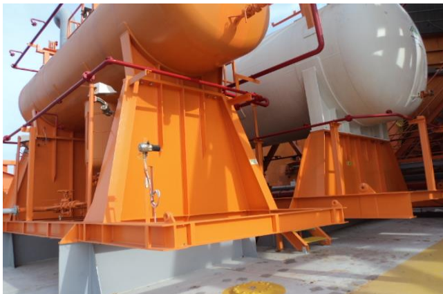
After final coat on P-40 & P-41area
