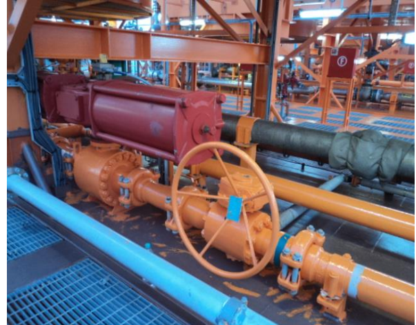
After final coat on top side of gas compressor area
