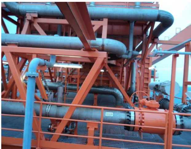
After final coat in P-10 top side
