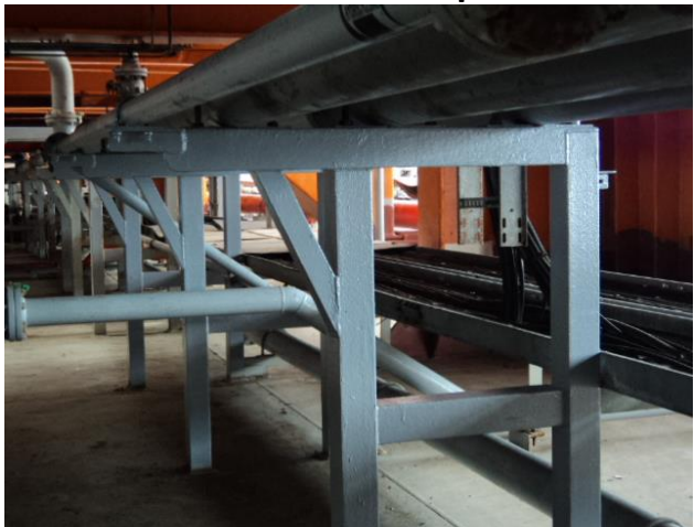
After final coat below main deck
