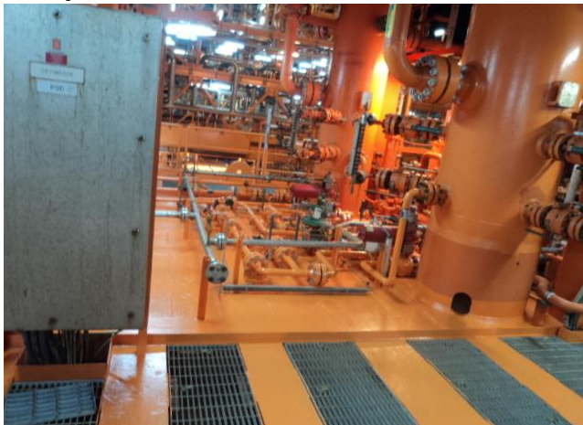
After final coat in gas compressor area
