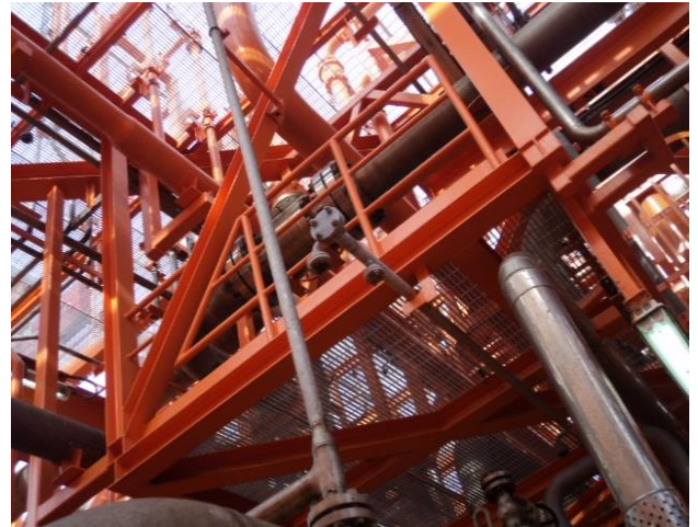
After final coat in P-10
