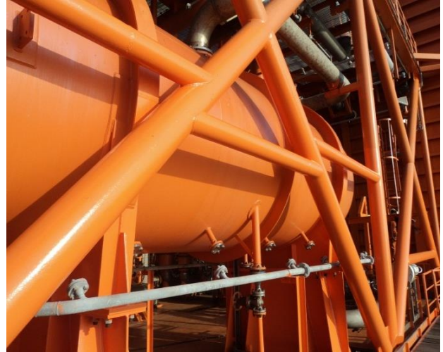
After final coat in P-10 area
