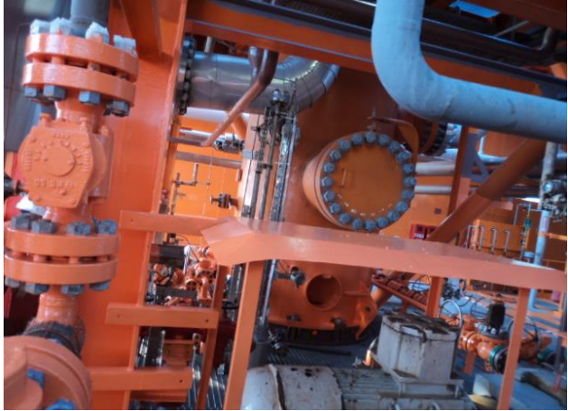
After final coat in U-71area
