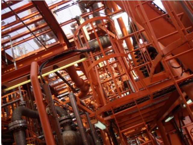
After final coat in P-11
