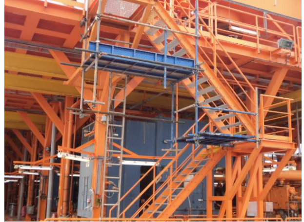
After final coat in Gas Compressor Area
